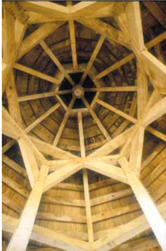
The headquarters of the Prince's Foundation is in the Shoreditch neighborhood of London's East End. This internal view shows a roof designed and constructed by students who attended the former Foundation Course. Photo courtesy of The Prince's Foundation.
